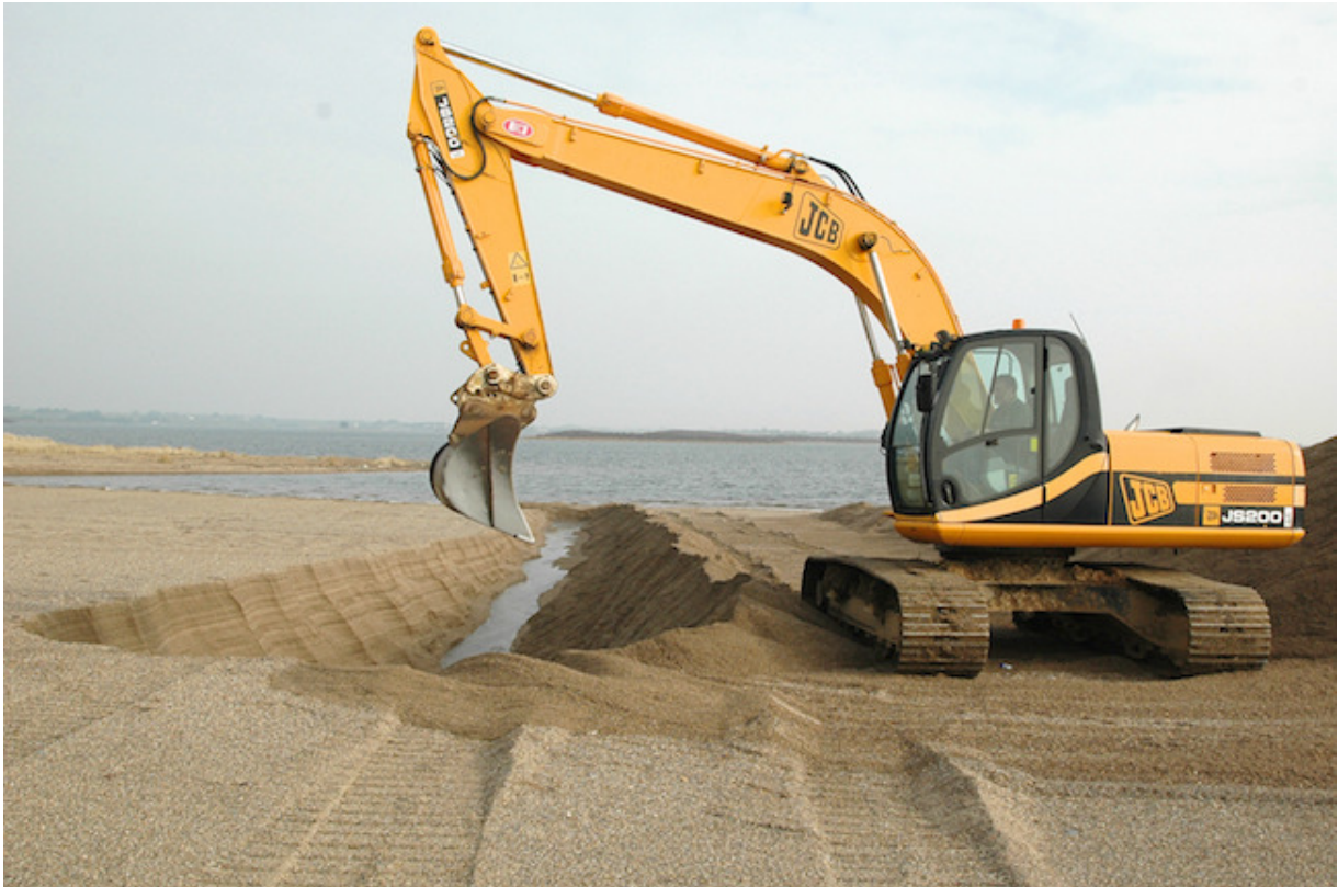
Breaching the barrier on 4 th March 2011.
